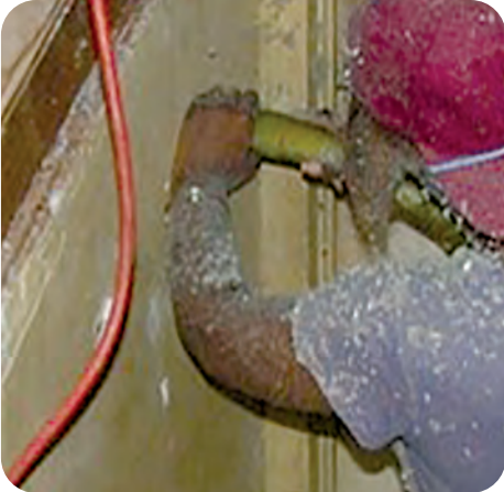
7. Dense pack stairway walls
