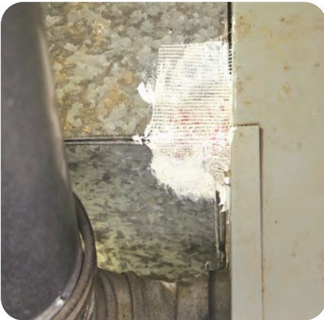
B-4. Push fiberglass mesh into the mastic
