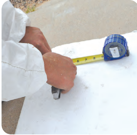
2. Cut blocking material to fit
