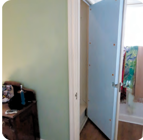
8. Weatherstrip and insulate door
