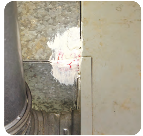
B-3. Apply mastic over the tape
