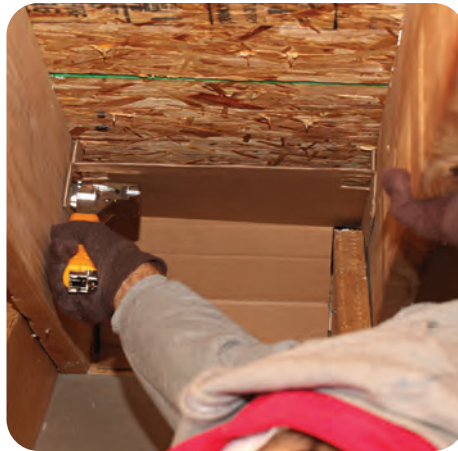
4. Install baffles at soffit vents if present. Ensure 1-2" vent space between baffle and roof deck for air flow. Baffles must extend a minimum of 6" beyond final insulation level.
