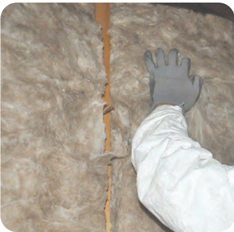
3. Install batts with minimal compression
